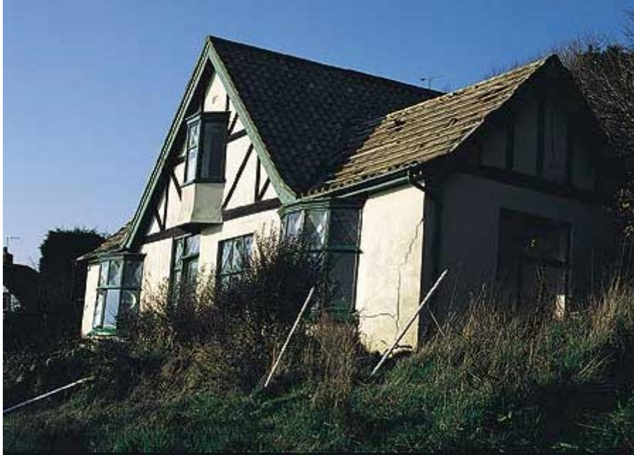
Plate G2b Property damage - Green Rooves, Luccombe (demolished (1988))
